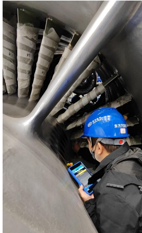
In the steam turbine assembly workshop, measure the gap between the rotor and the cylinder block
